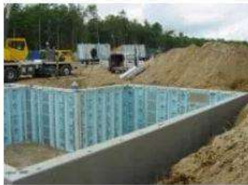
Figure 78 Precast Concrete Foundations
